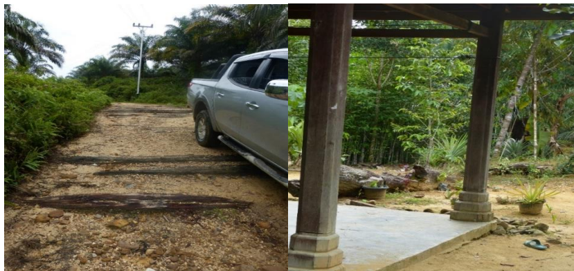
Figure 26 - Log of Merbau ( Intsia sp ) used for road (left) and building (right) construction
