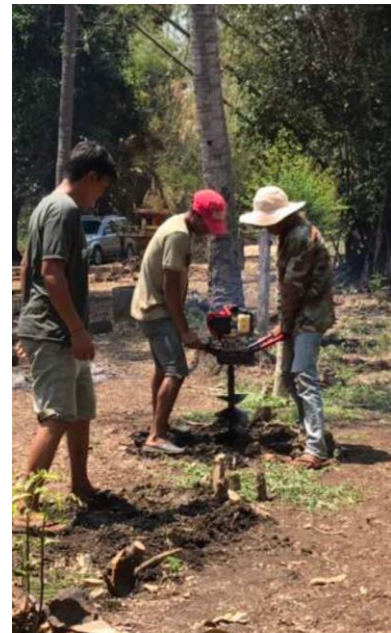
Figure 35 - Mechanical hole digger used for the installation of posts.
