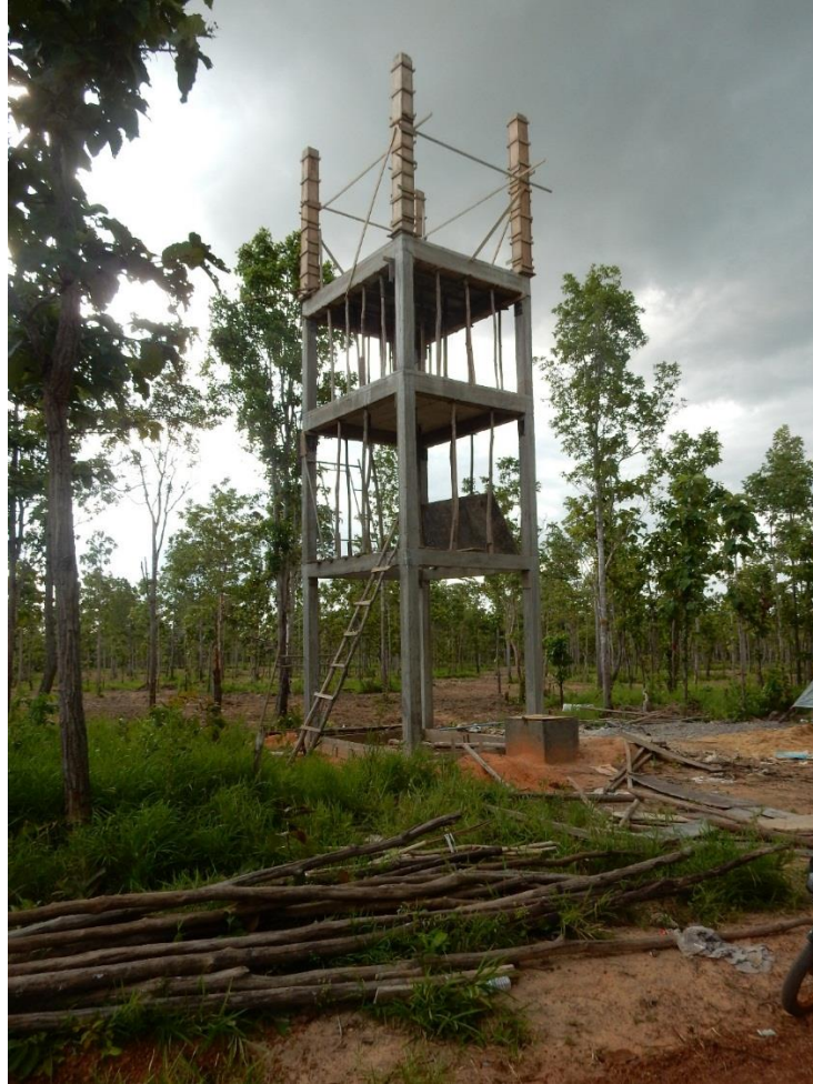
Figure 41. On-going construction of water tank in Ou Baktra CF
